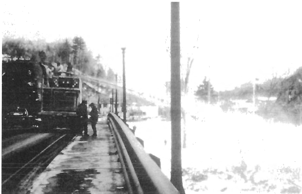
Figure 6. Hydroseeder being used to put leaves on the White River in Hartford, Vermont.
