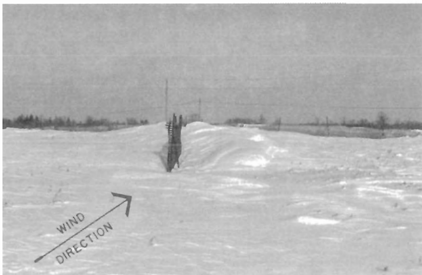
Figure 12. Snow Accumulations at Misaligned Fence
