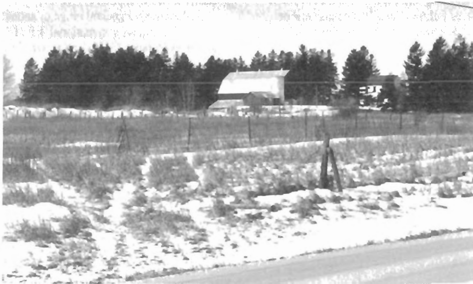
Figure 1. The fence in this example is not collecting snow because of a small upwind fetch and ground cover that will contain most driftable snow. There is not likely a severe problem at this site. The discontinuation of the use of this fence will not affect snow accumulation on the road and save in the order of $500 annually.
