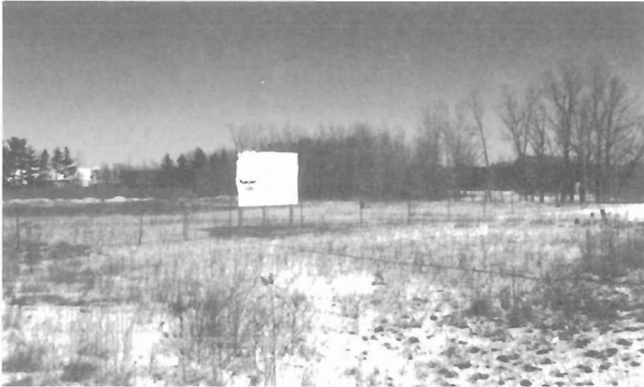
Figure 2. In this case the fence material used is intended for crowd-control and is not dense enough for snow fencing. The problem should be evaluated and if the severity warrants, install a fence with higher density. In this case $500 was wasted because an ineffective fence was installed. Opaque material (center) was used in this photo on billboard.
