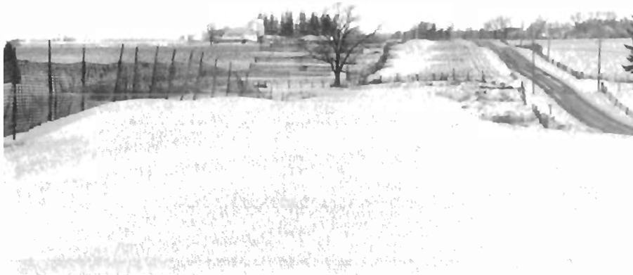
Figure 10. Recommended Solution - 2 Rows of snow fence
