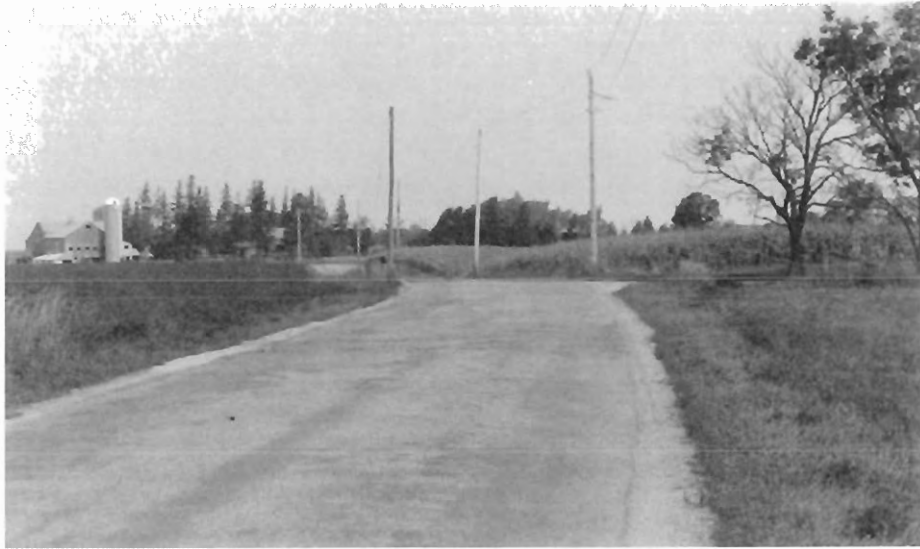
Figure 6. Woolwich Street Site - Waterloo
