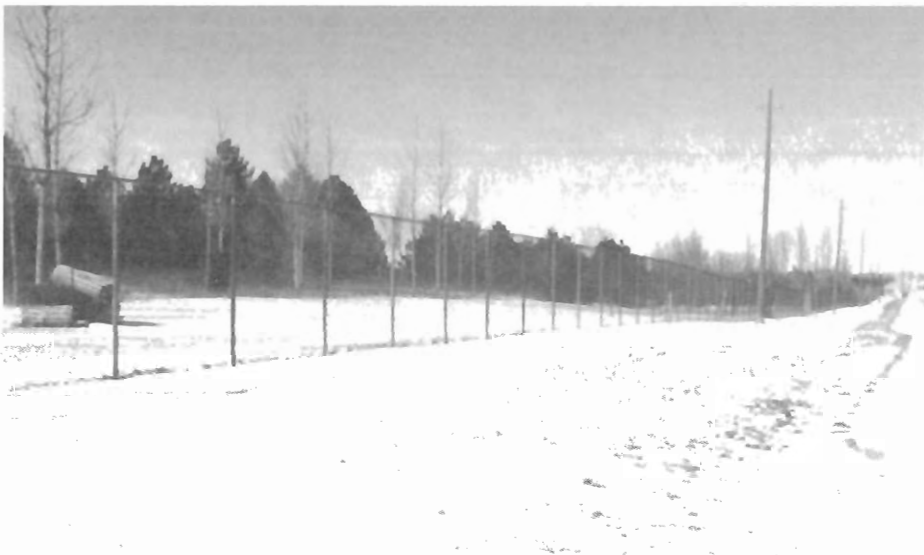
Figure 3. The discontinuation of the use of snow fencing at this site in favour of a permanent row of trees eliminates the annual installation of fencing. Annual savings for 300m of the road shown could be $1,500 .
